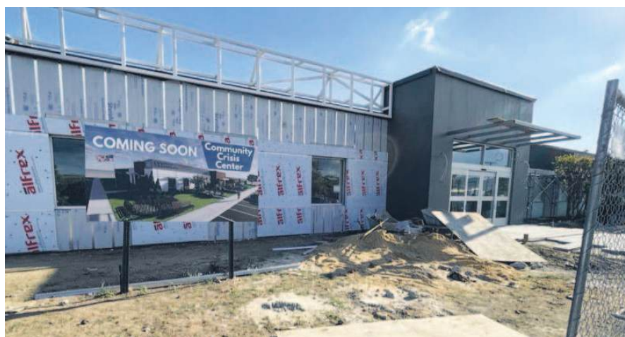
CN Guidance upcoming crisis center construction site.
